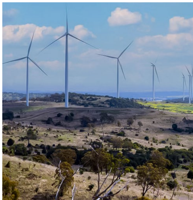
Image courtesy of Powerlink.
