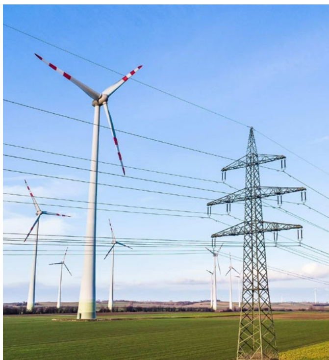
Image courtesy of Powerlink.
